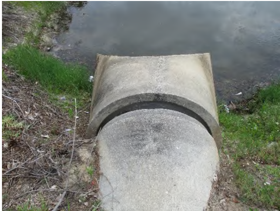
SW corner pipe separation
