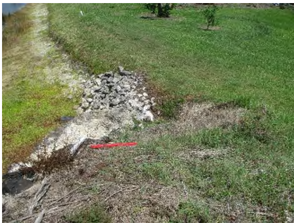
SW corner erosion and washout.
